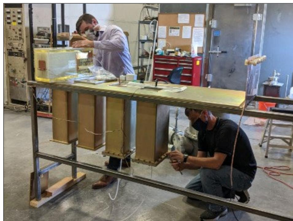
Figure 2. Graduate student Travis Bejines and IAC Engineer Brian Berls assembling the 4-Brick Cinco generator. This device, capable of 320 kA, will allow the validation of all key components, a necessary step before building larger Cinco devices with ramp compression loads.
